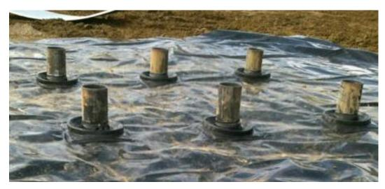
A common design feature of any secondary containment system is the use of posts or pilings to support the tank that will be providing the primary containment. However when this construction technique is utilized, at issue is how to best attach the geomembrane liner to any pilings that now penetrate the geomembrane liner.
